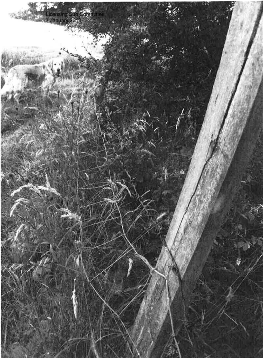
DAMAGED STOCK FENCE IN FIELD BELONGING TO HIGH TREES COTTAGE
